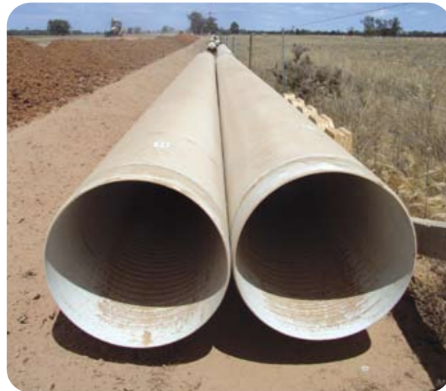
Photo: Glass reinforced plastic pipe being laid south of Donald
