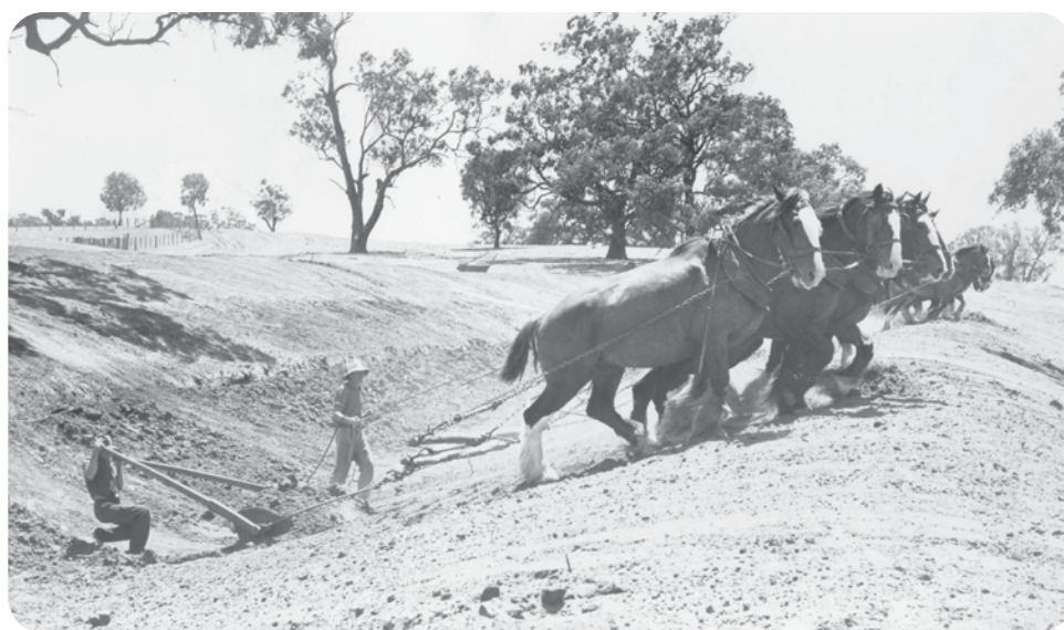
This historic photograph shows Clydesdale horses and Wimmera pioneers building Toolondo channel, which is part of the Wimmera Mallee stock and domestic open channel system. This photograph was taken about 20 kilometres south of Horsham in the mid to late 1950s.
